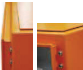
Closeup photo of gutter and welding detail
