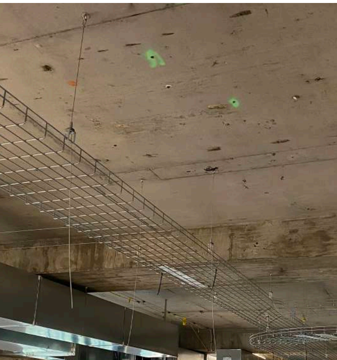
Cable basket adaptor installations
