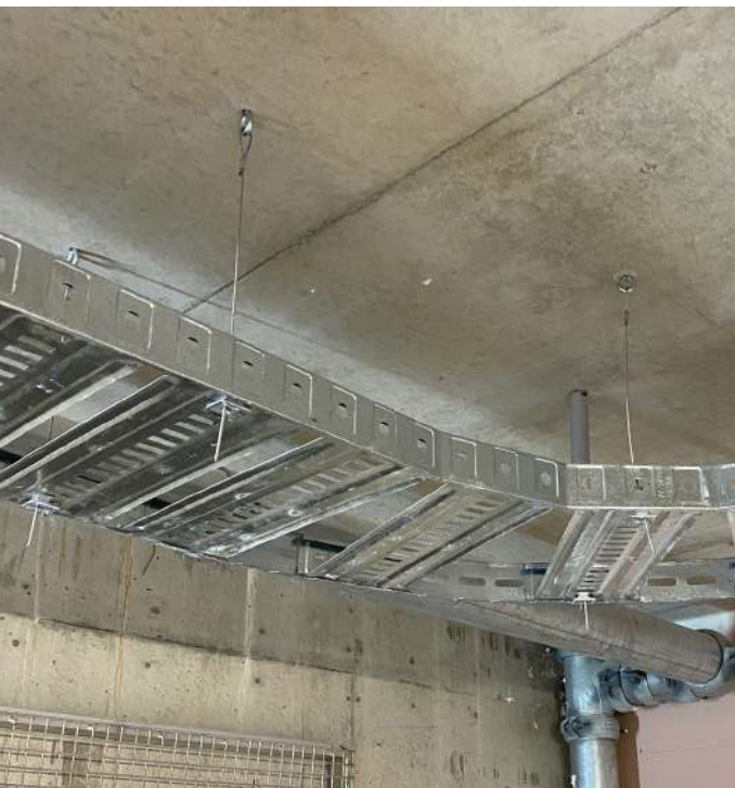
Installation without strut
